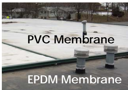
Photo of roof on December 15, 2003
