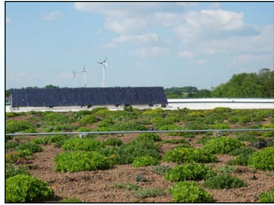
Prairie Green Roof System
