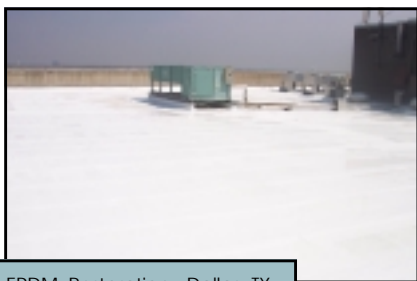
EPDM Restoration - Dallas, TX
