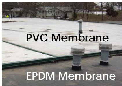
Photo of roof on December 15, 2003
