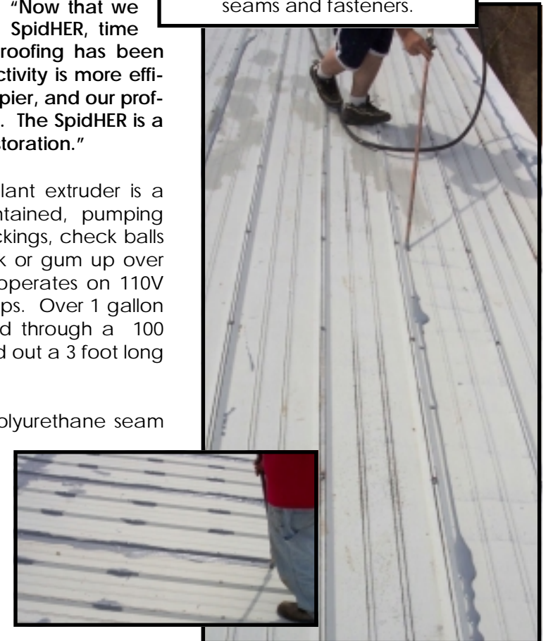
The SpidHER at work sealing seams and fasteners.
