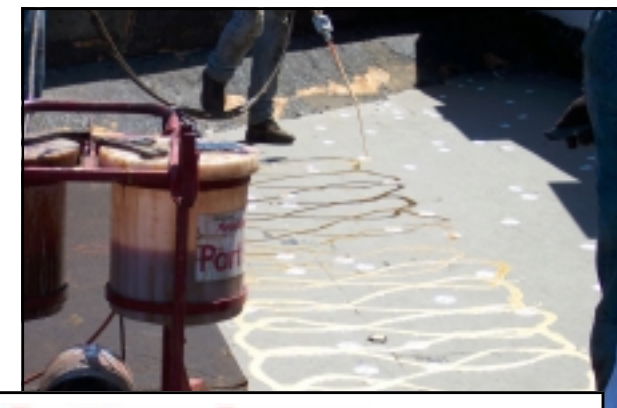
OlyBond 500 in action with the PaceCart applying a tapered insulation system in Iowa.
