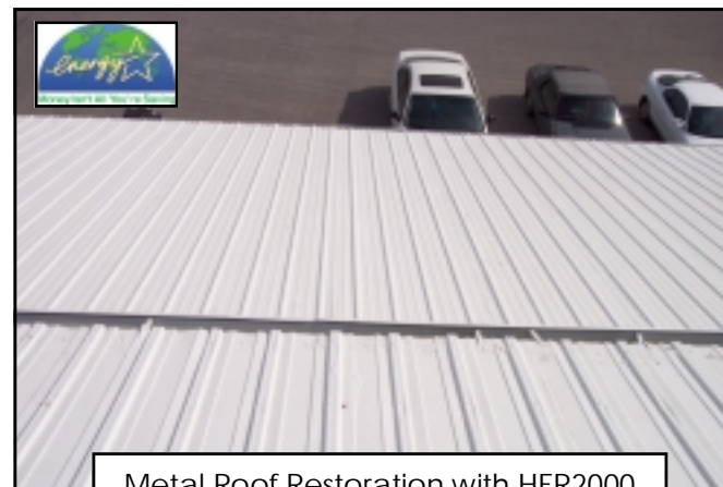
Metal Roof Restoration with HER2000 over seams and fasteners and Era-guard 1000 Acrylic Top Coat
