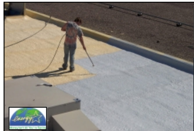
Spray Polyurethane Foam with Erathane 300 Base Coat and Erathane 300 Finish Coat
