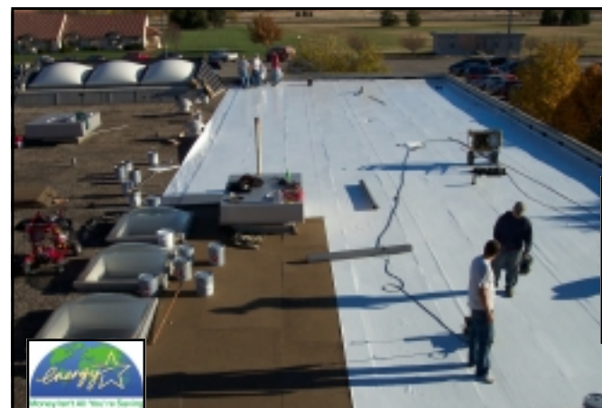
Metal Roof Restoration with HER2000 over seams and fasteners and Era-guard 1000 Acrylic Top Coat
