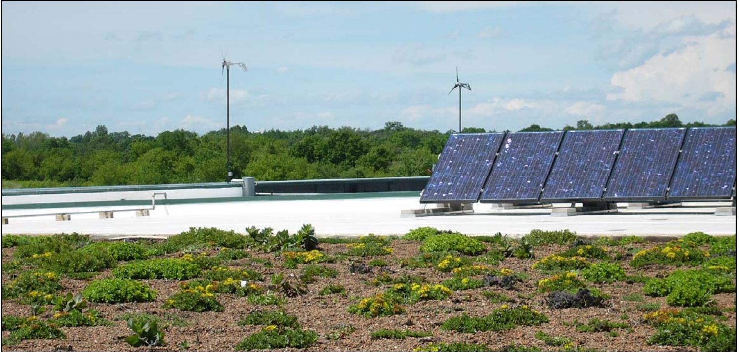
Photo shows Prairie Green Roof System in Foreground with Solar Panels on Right and Small Scale Wind Turbines on Left
