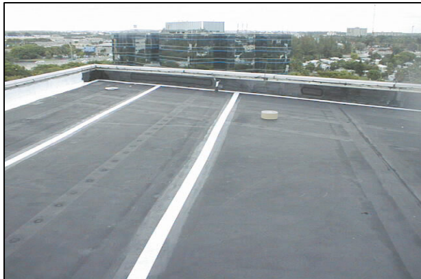
Photo of EPDM Restoration (in progress) with EG1000 Acrylic on the left and Smooth Modified Asphalt Restoration Combining Erathane Ultra Water Based Polyurethane and ERLASTIC Acrylic on the right
