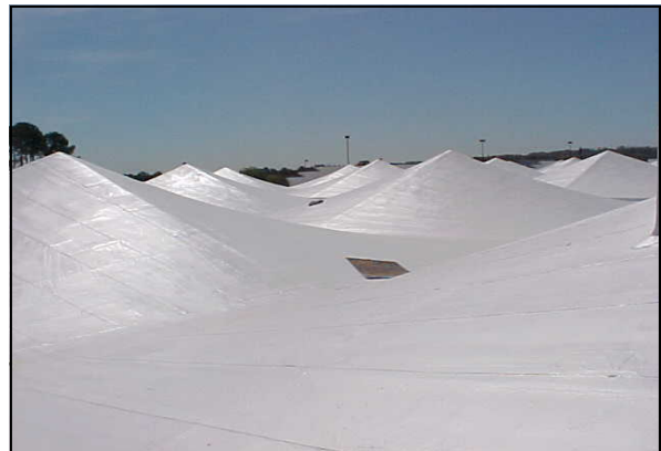
Photo of EPDM Restoration (in progress) with EG1000 Acrylic on the left and Smooth Modified Asphalt Restoration Combining Erathane Ultra Water Based Polyurethane and ERLASTIC Acrylic on the right
