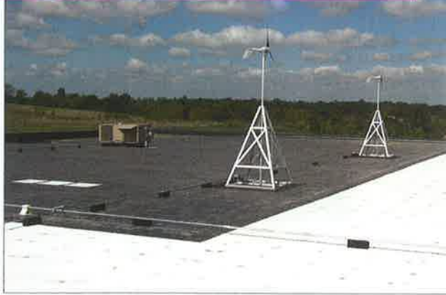
An infrared scan shows the lower temperature of the coated portion of this EPDM roof.
